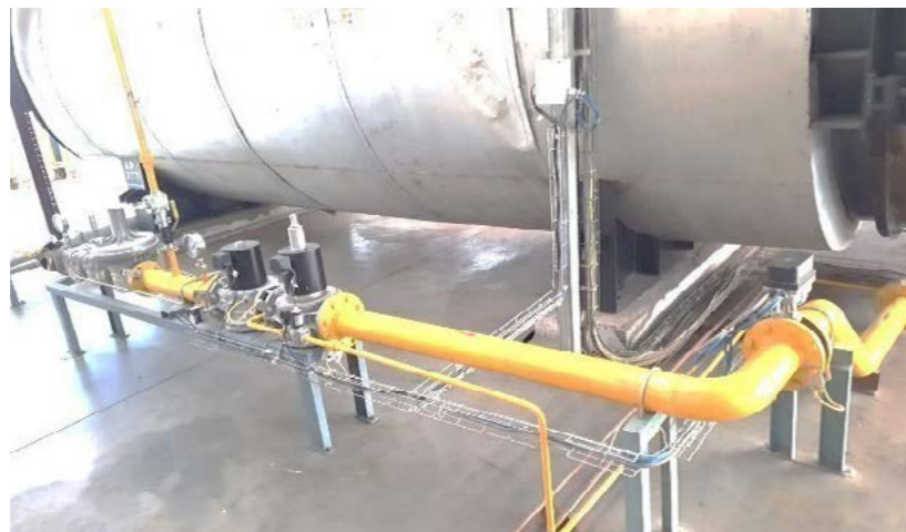
Boiler fuel conversion from HSD to PNG
